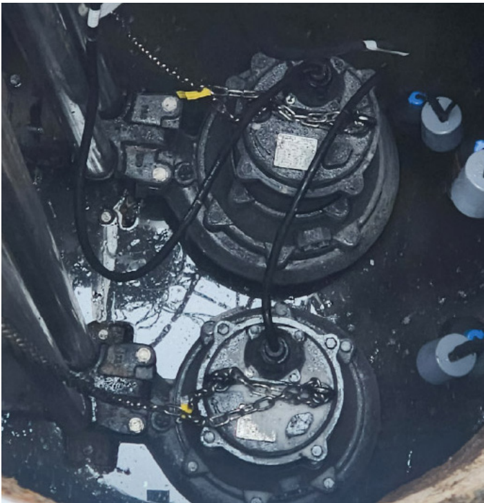
Tsurumi's products operating reliably in a demanding dewatering environment.
